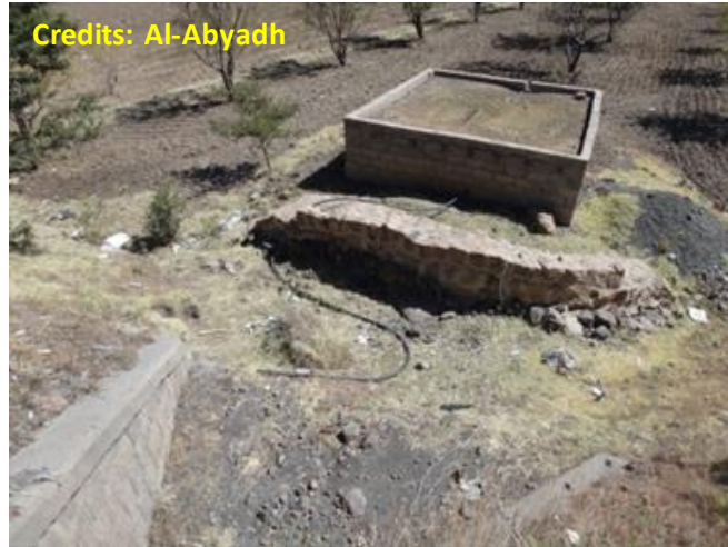
Photo 2.37 Erosion Control at culvert outlet by using semi-circular stone masonry wall
