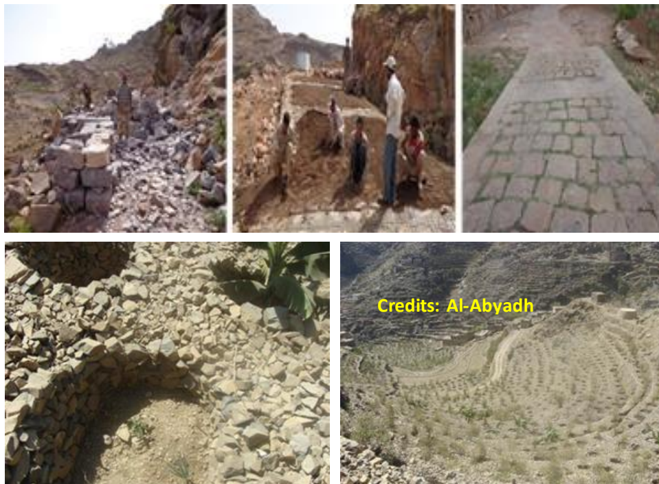
Photo 4.6 Stone mulching from local quarry material by using the access rock from rock shaping which used to pave rural roads
