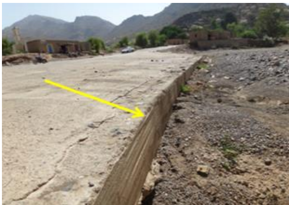
Photo 2.15 Scour of wadi Hamidha ( Al-Mahweet gov.) irish crossing structure due to the huge seasonal floods and the extended protection works
