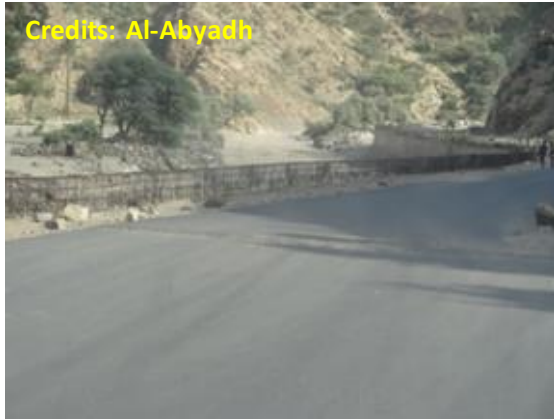
Photo 2.43 Erosion protection reinforced concrete wall when the road embankment pass near water course (wadi)
