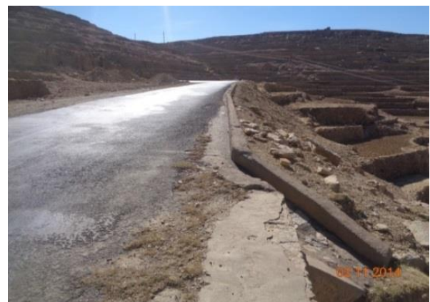
Photo 2.36 Erosion Control at side shoulder embankment using lined spillway(left) and controlled road run-off using curb barriers and spillway (right)
