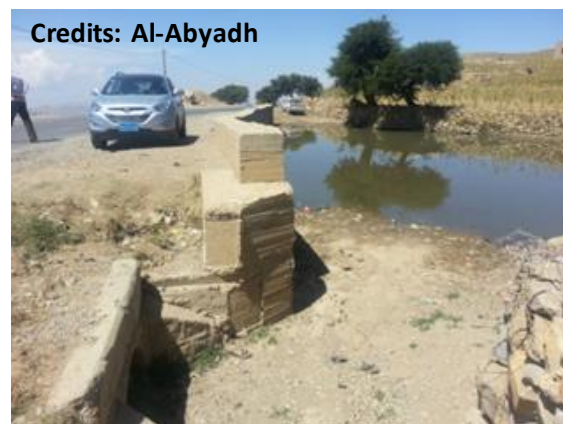
Photo 3.4 Direct storage using the protection cyclopean concrete wall and by closing the culvert inlet
