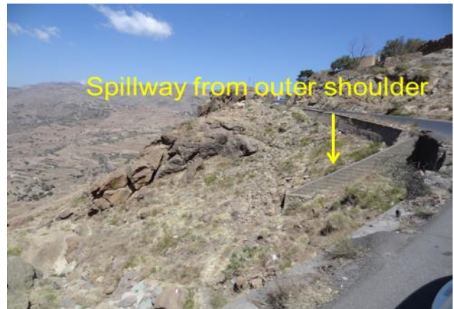
Spillway from up-slope and from outer shoulder along retaining wall, photos credits: Al-Abyadh
