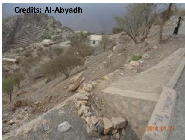
Photo 3.5 Harvested runoff directed to the storage system using catch basin and polyethylene pipe from culvert outlet
