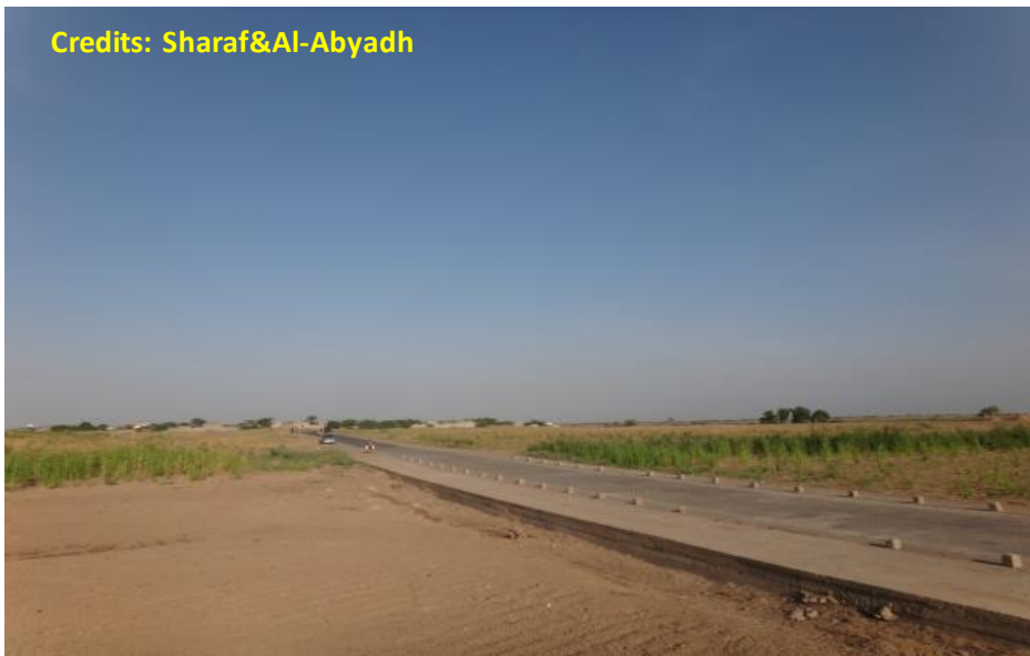
Photo 2.13 Example of irish crossing in flat terrain
