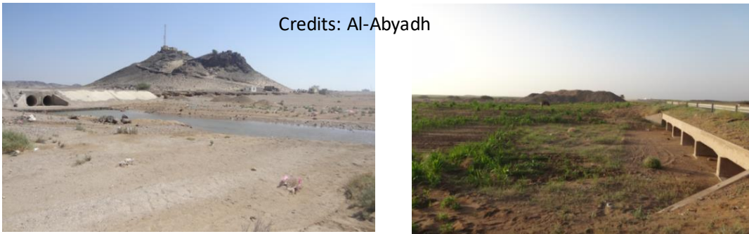
Photo 2.12 Culvert in costline and flat area
