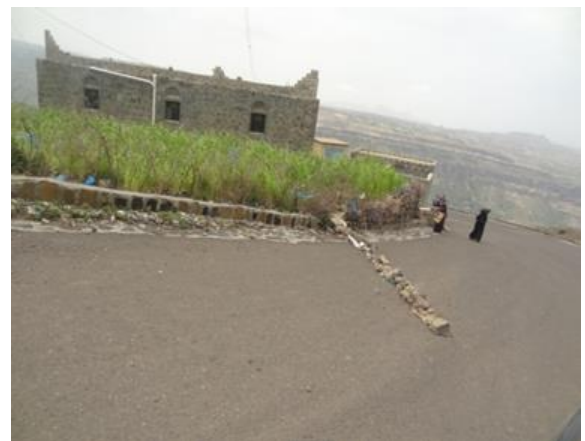
Photo 3.13 Runoff is directed to storage ponds or underground cisterns using catch basins and underground pipes (left), and runoff is directed to irrigated farms using temporary humps (right)
