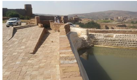
Photo 1.3 Reservoirs constricted in middle areas between houses to harvest rainwater from roofs & surrounding areas
