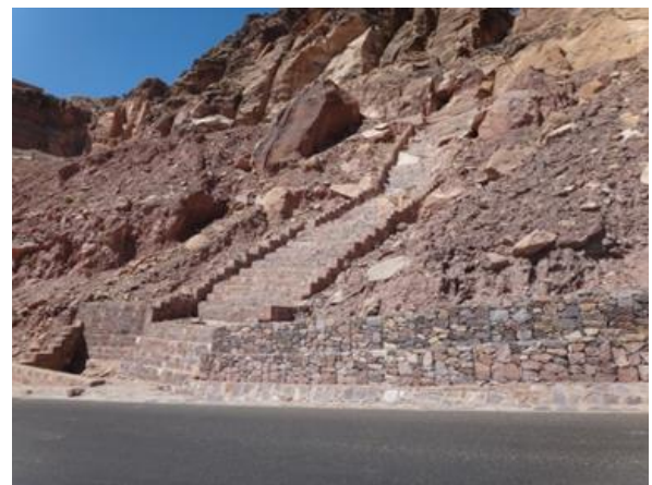
Photo 2.41 Erosion Control at culvert Inlet using gabions walls & Erosion Control at cut side of the culvert outlet using gabions walls and erosion protection riprap cascade spillway
