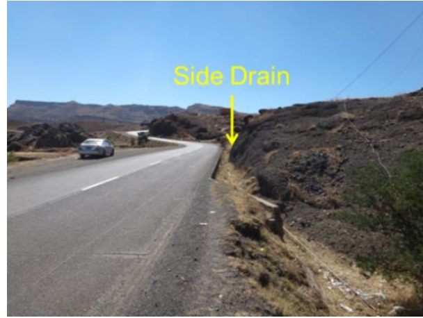
Photo 2.18 Side drains and lead out drain (mitre drain)
