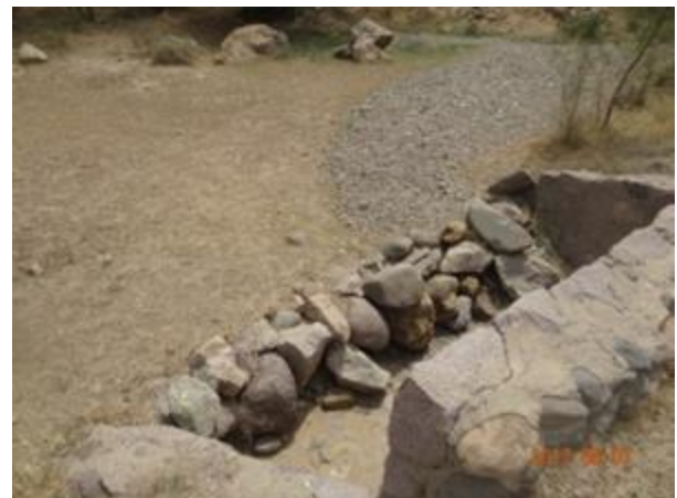
Photo 2.39 Erosion control at culvert outlet/inlet by using dry stone check wall
