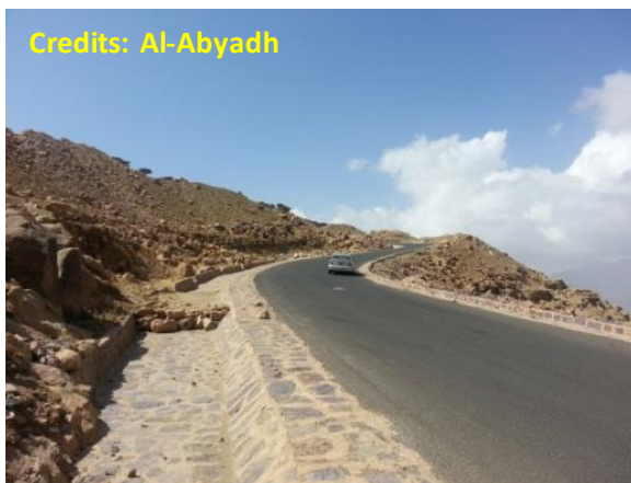
Photo 2.42 Temporary rock scour checks in a rip-rapped side ditches
