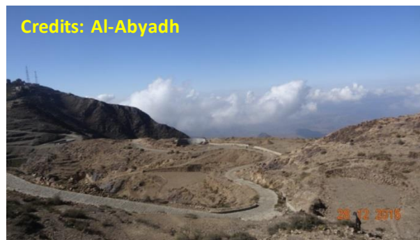
Photo 3.10 common road surface drainage method
