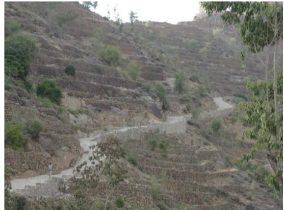
Photo 3.15 Direct irrigation from road surface and water harvested from side curbs / barrier
