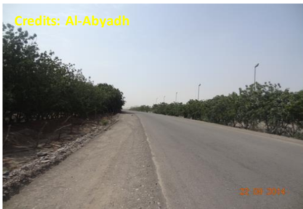
Photo 4.8 Road side plantation in flat areas may protect the road embankment from erosion
