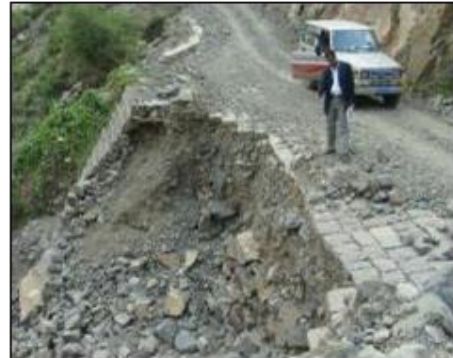
Photo 2.1 Runoff inside Drainage and Cross Drainage Damage in Yemen
