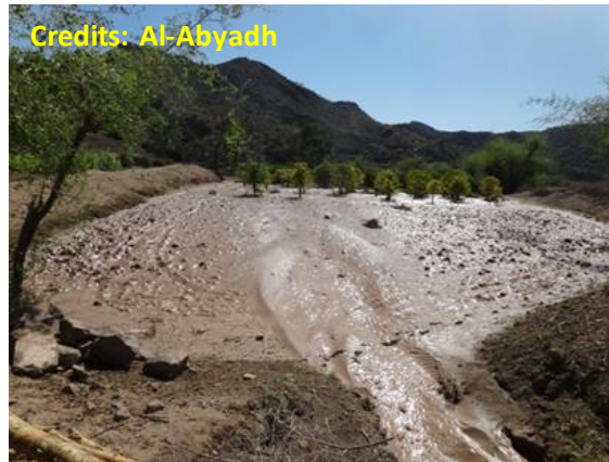
Photo 4.3 Culverts and hump leads runoff water to storage reservoirs, recharge structures or directly to land
