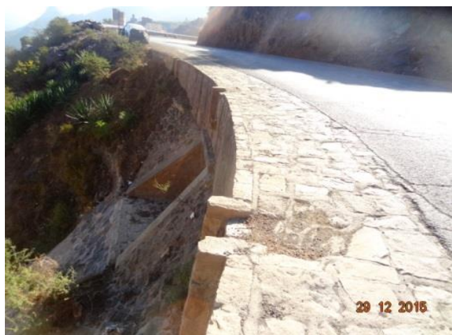
Spillway at the retaining wall and cascade spillway at the culvert outlet, photos credits: Al-Abyadh
