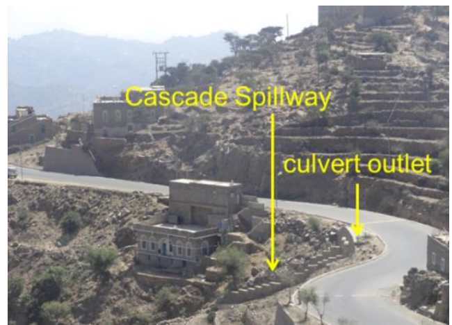
Spillway at the retaining wall and cascade spillway at the culvert outlet, photos credits: Al-Abyadh
