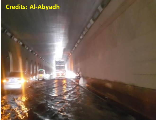
Photo 3.39 Water tunnel tanks may act as harvesting structure temporarily
