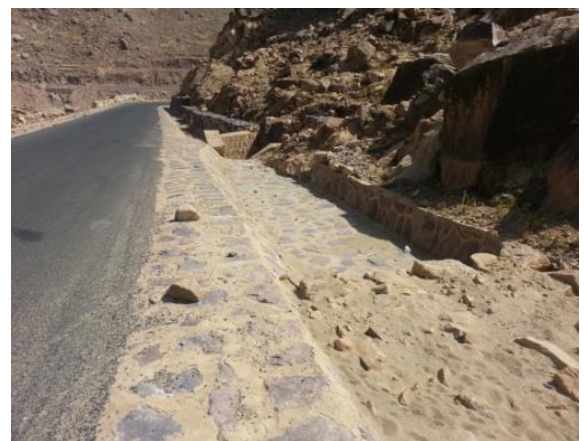
Photo 2.42 Temporary rock scour checks in a rip-rapped side ditches
