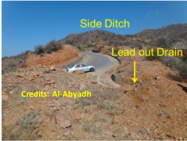
Photo 2.18 Side drains and lead out drain (mitre drain)
