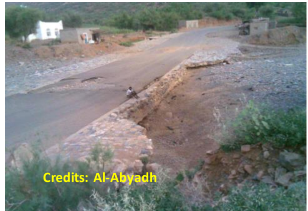
Photo 2.14 Show the sedimentation problem on arch bridge
