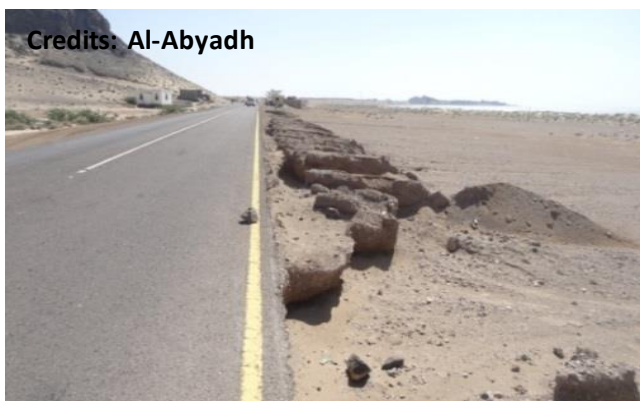
Photo 2.29 Erosion at side shoulder and embankment
