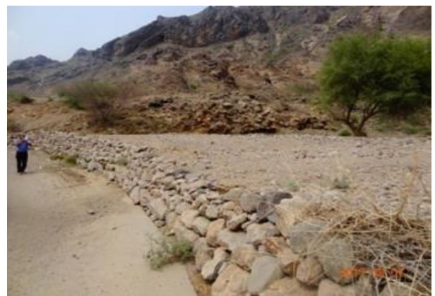
Photo 2.45 Scour and debris control at irish crossing using dry check stone wall at the upstream side of the water course. It minimizes the accumulation of debris materials along the road surface and reduce the scour effect at the outlet
