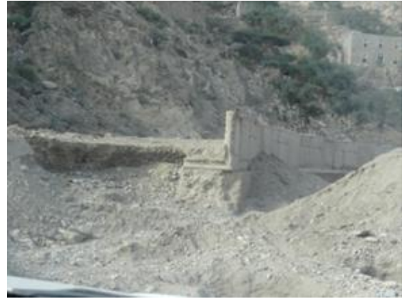
Photo 2.43 Erosion protection reinforced concrete wall when the road embankment pass near water course (wadi)
