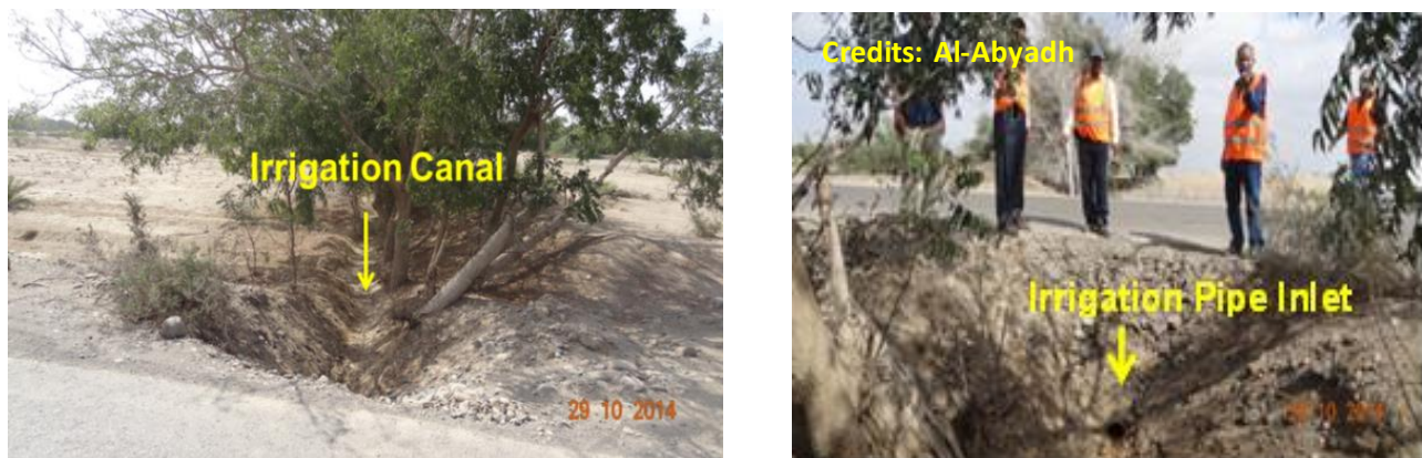
Photo 2.22 Small Plastic pipe used for irrigation purposes
