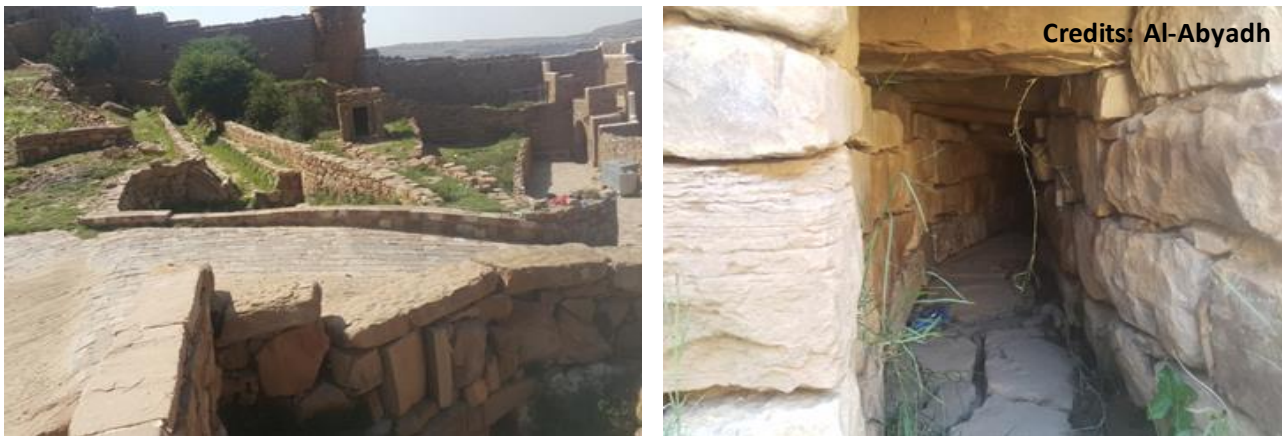
Photo 1.5 Canal under stone paved road to convey rainwater to cisterns
