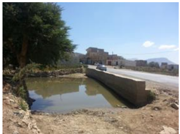
Photo 3.4 Direct storage using the protection cyclopean concrete wall and by closing the culvert inlet
