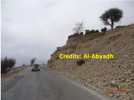
Photo 4.7 Road side plantation will act as soil stabilization and mitigate landslide of the road slopes in mountain areas
