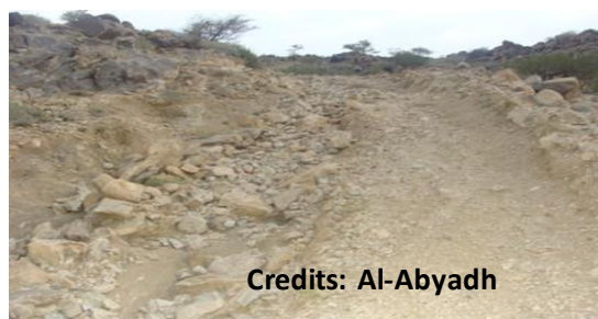
Photo 3.30 Earthen roads risk developing into a flood path – proper design with rolling dips and spill overs required
