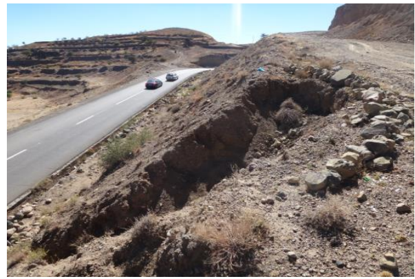
Photo 2.27 Erosion at road cut section
