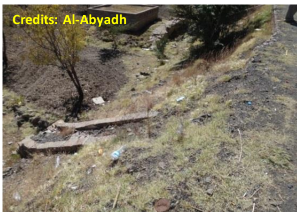
Photo 2.36 Erosion Control at side shoulder embankment using lined spillway(left) and controlled road run-off using curb barriers and spillway (right)
