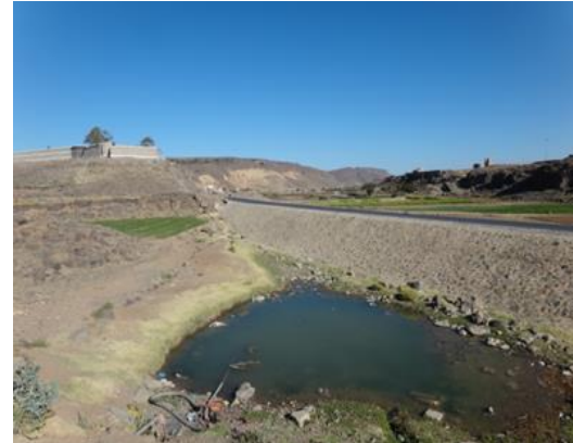
Photo 3.22 Road embankment used as water harvesting body with riprap protection works
