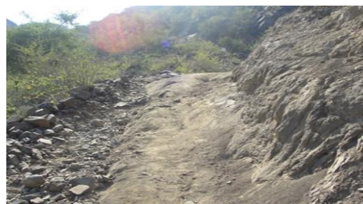
Photo 3.30 Earthen roads risk developing into a flood path – proper design with rolling dips and spill overs required
