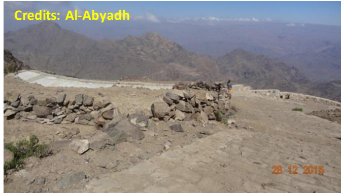
Photo 3.11 Earth hump as road surface drainage methods
