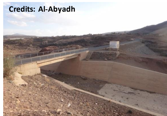
Photo 3.20 Road body used as recharge dam in asphalt road
