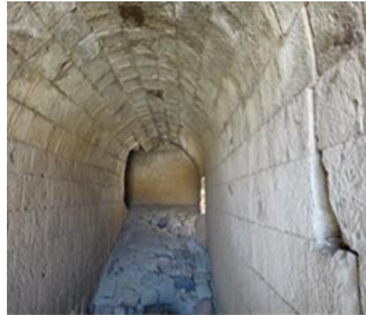
Photo 2.23 Water diversion culvert with 90° angle to cope water rights issues
