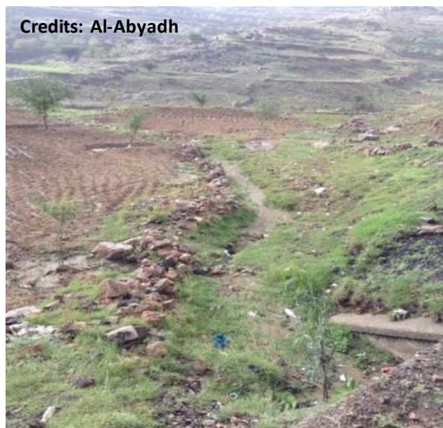
Photo 3.2 Indirect diversion from culvert outlet using earth channel to Almonds farm
