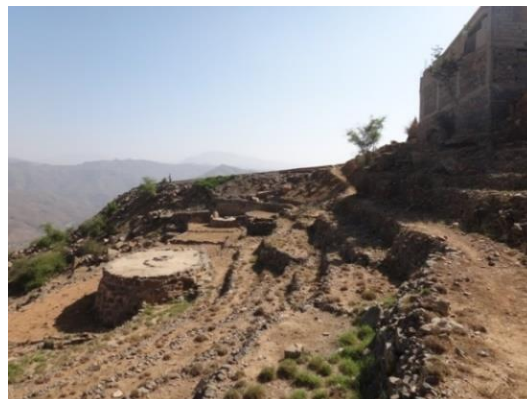
Photo 3.8 Cistern filled from road recharge and stone blocking first flush, Al Wastah
