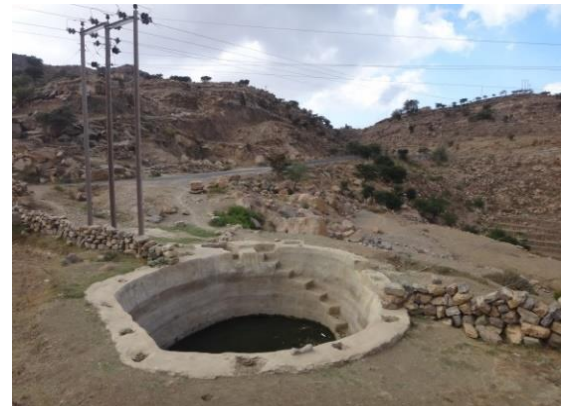
Photo 3.6 Ponds harvesting water from side drains
