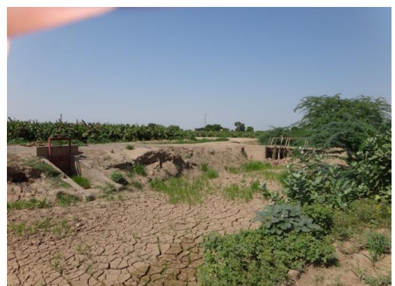
Photo 2.47 Using the Culverts provided with control gates in Wadi Zabid to facilitate distribute floods in sub-canals
