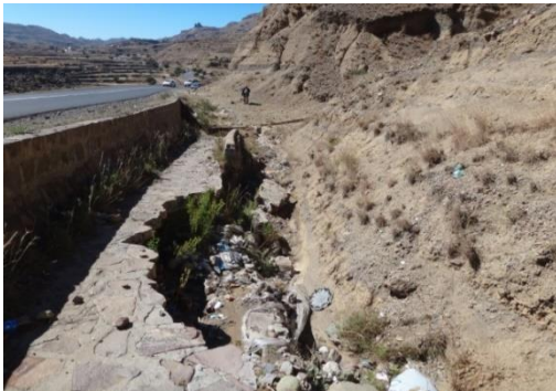
Photo 2.1 Runoff inside Drainage and Cross Drainage Damage in Yemen
