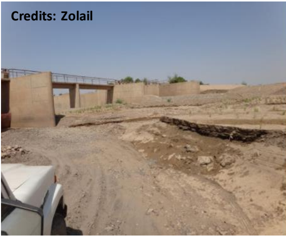
Photo 2.46 Using the bridges in Wadi Zabid to facilitate the floods movement in main-canals
