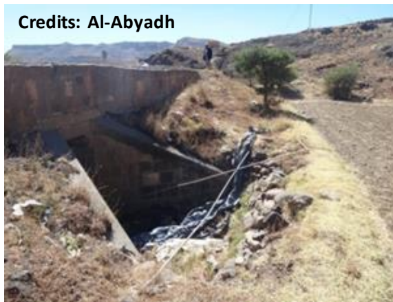
Photo 2.39 Erosion control at culvert outlet/inlet by using dry stone check wall
