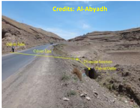
Photo 2.23 Water diversion culvert with 90° angle to cope water rights issues
