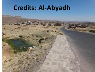
Photo 3.27 Road embankment (left), interferes with base subsurface spring flow; the intercepted water appeared on the other side (middle picture), the spring flow point (right)
