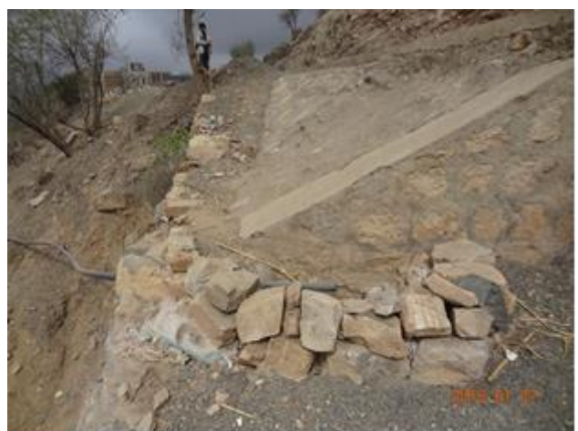
Photo 3.5 Harvested runoff directed to the storage system using catch basin and polyethylene pipe from culvert outlet
