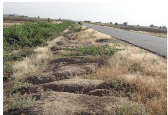
Photo 2.29 Erosion at side shoulder and embankment
