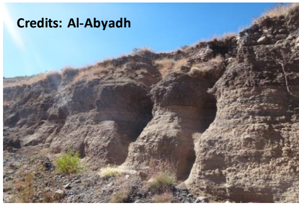
Photo 2.27 Erosion at road cut section
