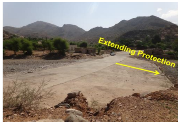
Photo 2.15 Scour of wadi Hamidha ( Al-Mahweet gov.) irish crossing structure due to the huge seasonal floods and the extended protection works
