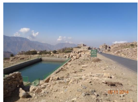
Photo 3.7 Road-run-off collected respectively from (up-slope) side drainage and from escape in down-slope side drain
