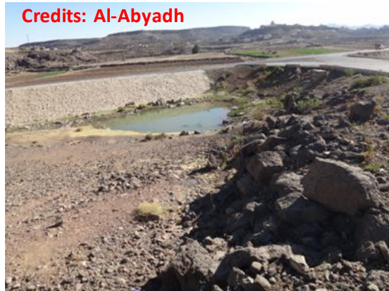
Photo 3.22 Road embankment used as water harvesting body with riprap protection works
