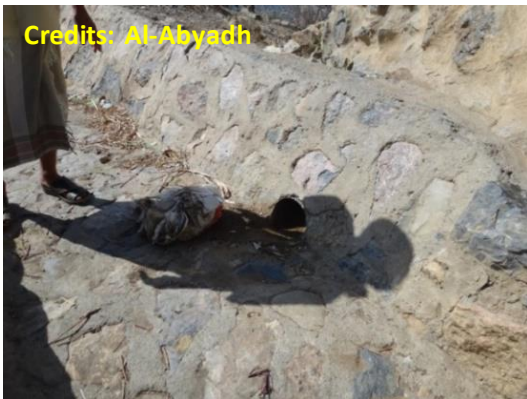
Photo 3.8 Cistern filled from road recharge and stone blocking first flush, Al Wastah
