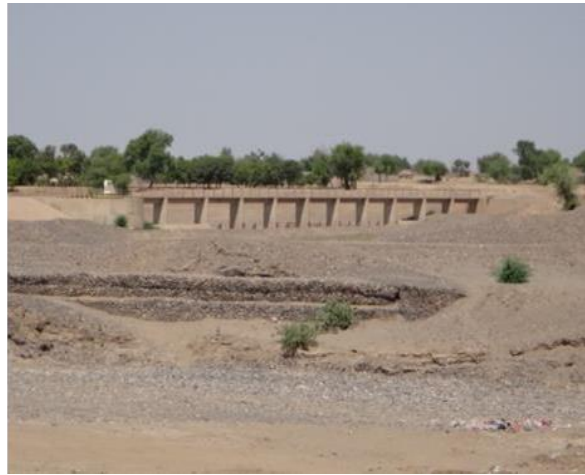
Photo 2.46 Using the bridges in Wadi Zabid to facilitate the floods movement in main-canals
