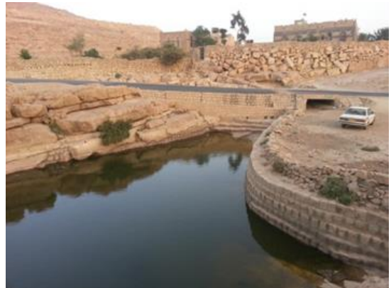
Photo 3.3 Direct storage at the culvert outlet
