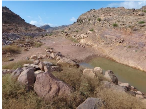
Photo 3.16 Using a borrow pit in Wadi Tabab near the road as retention and recharge pond (left)
