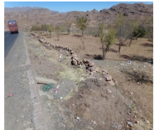
Photo 2.38 Erosion Control at culvert Inlet by using Sand bag to control the flood and the Outlet by using dry stone wall and earth longitudinal canal
