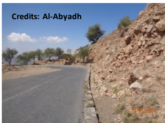
Photo 3.7 Road-run-off collected respectively from (up-slope) side drainage and from escape in down-slope side drain
