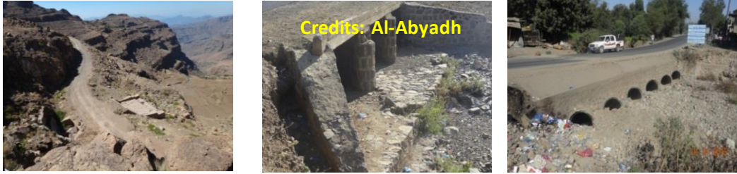
Photo 2.11 Culverts in mountains area
