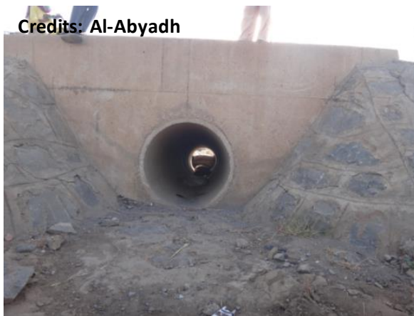
Photo 2.38 Erosion Control at culvert Inlet by using Sand bag to control the flood and the Outlet by using dry stone wall and earth longitudinal canal
