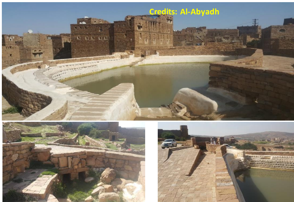
Photo 1.3 Reservoirs constricted in middle areas between houses to harvest rainwater from roofs & surrounding areas
