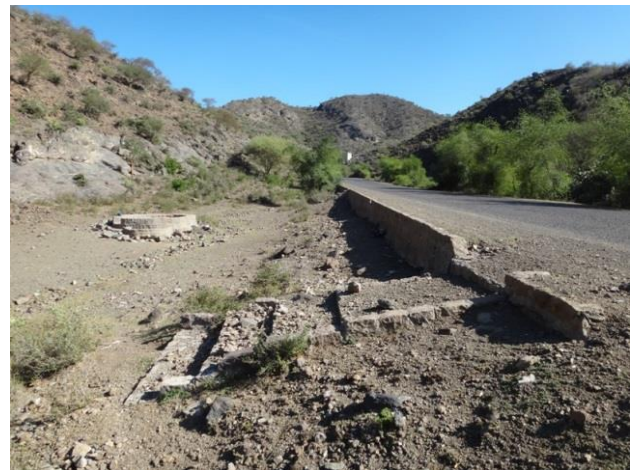
Photo 3.12 Flood water guider from roads (left) and stepped intake (right)
