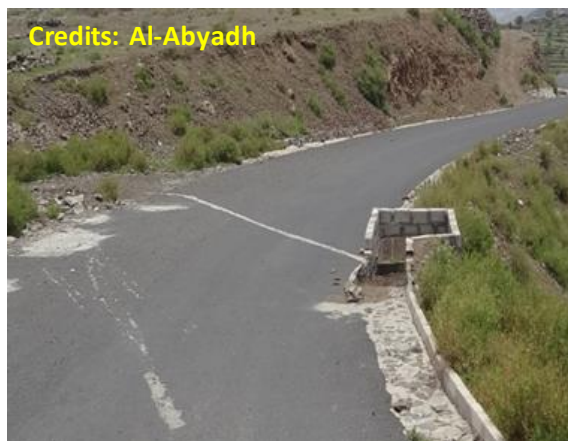
Photo 3.13 Runoff is directed to storage ponds or underground cisterns using catch basins and underground pipes (left), and runoff is directed to irrigated farms using temporary humps (right)
