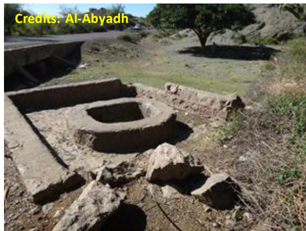
Photo 4.11 Recharge of hand-dug wells near culvert outlet in water stream
