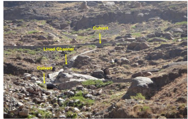
Photo 2.40 Erosion control using lined channel between culverts in mountains area
