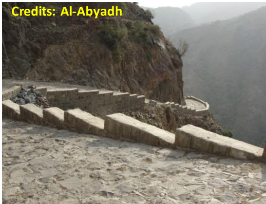
Photo 3.15 Direct irrigation from road surface and water harvested from side curbs / barrier
