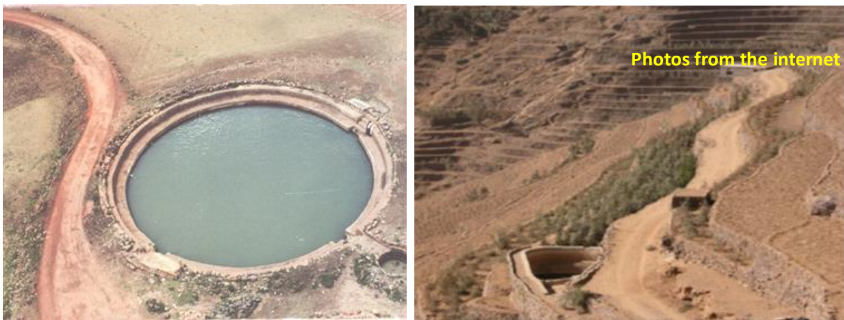
Photo 1.6 Rainwater harvesting from roads surface and drainage
