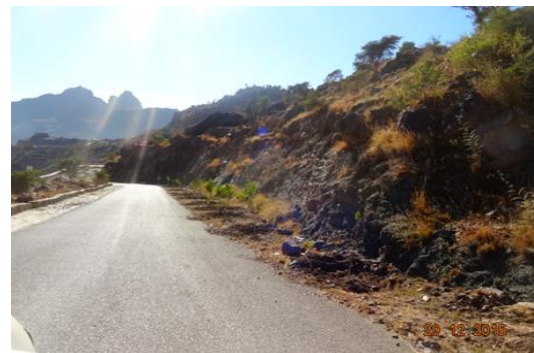
Photo 3.23 Road side plantation using semi arch bunds in the road shoulder in mountainous areas
