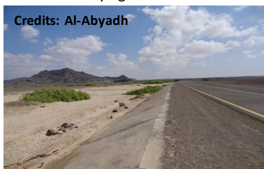
Photo 3.29 The embankment was protected by concrete and there is a small temporary bund to retain the water in the upstream (the potential is using gates in the culverts inlets)
