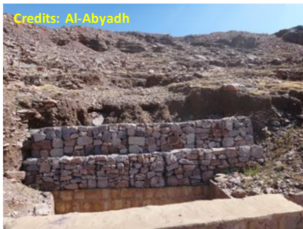
Photo 2.41 Erosion Control at culvert Inlet using gabions walls & Erosion Control at cut side of the culvert outlet using gabions walls and erosion protection riprap cascade spillway
