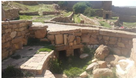
Photo 1.3 Reservoirs constricted in middle areas between houses to harvest rainwater from roofs & surrounding areas
