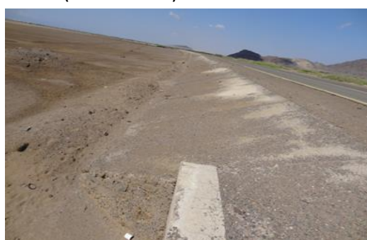
Photo 3.29 The embankment was protected by concrete and there is a small temporary bund to retain the water in the upstream (the potential is using gates in the culverts inlets)
