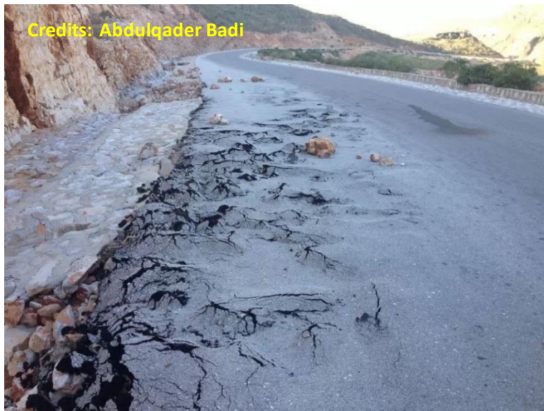
Photo 2.35 Pavement failure in Mori – Daksam road (Socotra island)
